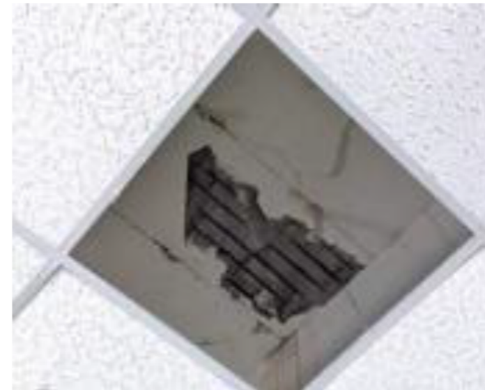
Examples of RAAC panel installation – not applicable to this site
