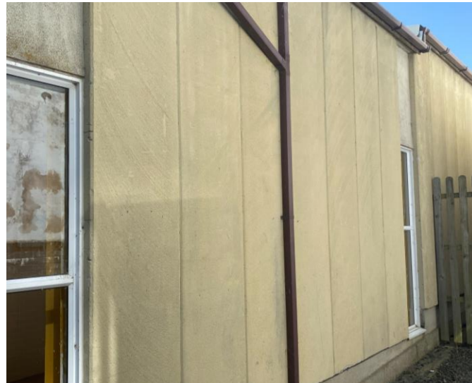
Form of Construction Photo 1 Elevation. Panelised construction
